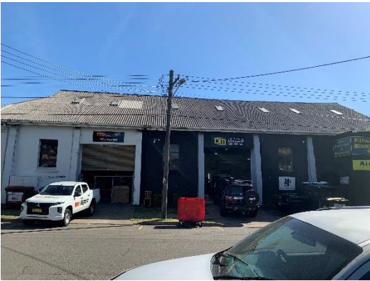
Empire Hall, south elevation.
