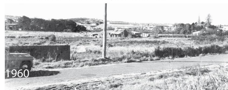
Future Warringah Mall site, Mynor factory visible at rear, trees at right surround Brookvale House
