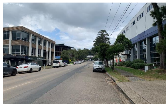
Figure 3.15 Industrial buildings along Old Pittwater Road.
